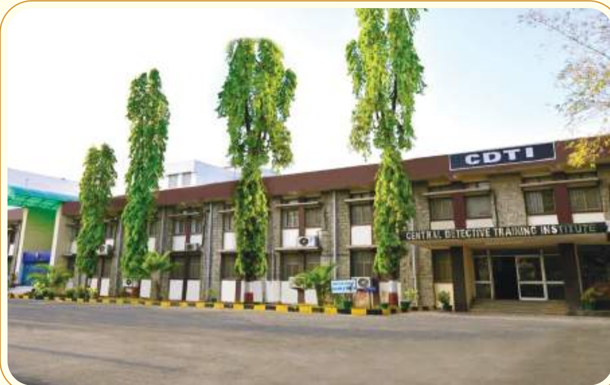
Front view of Admin building of CDTI, Hyderabad
